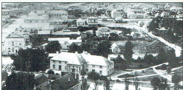
View over the business area from Onslow Road, 1876
