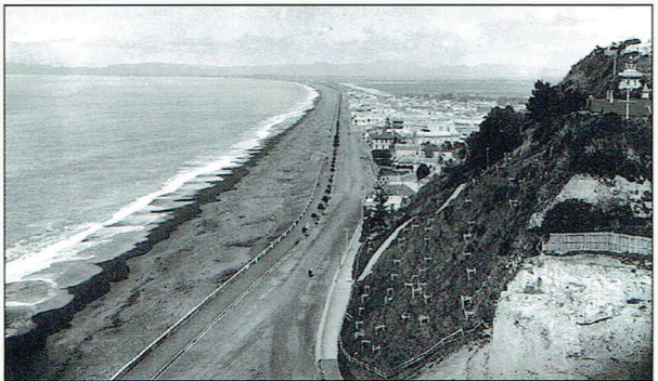
The prison and Marine Parade c1890. Construction of the sea wall and the roadway is taking place.
